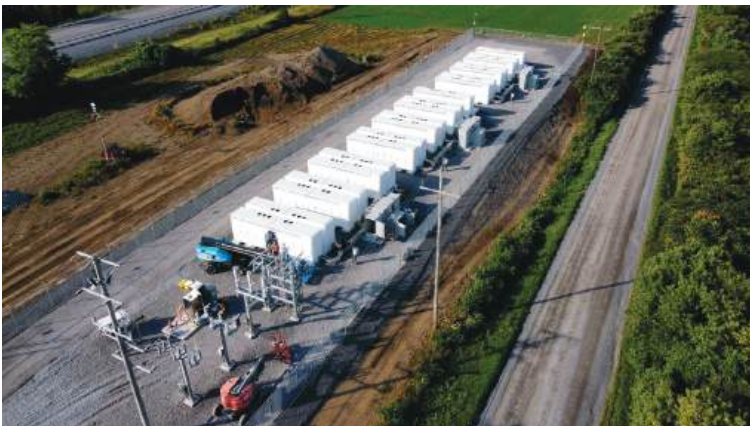
Photo – North Glengarry BESS (16.3MWac) nears mechanical completion – September 2025
